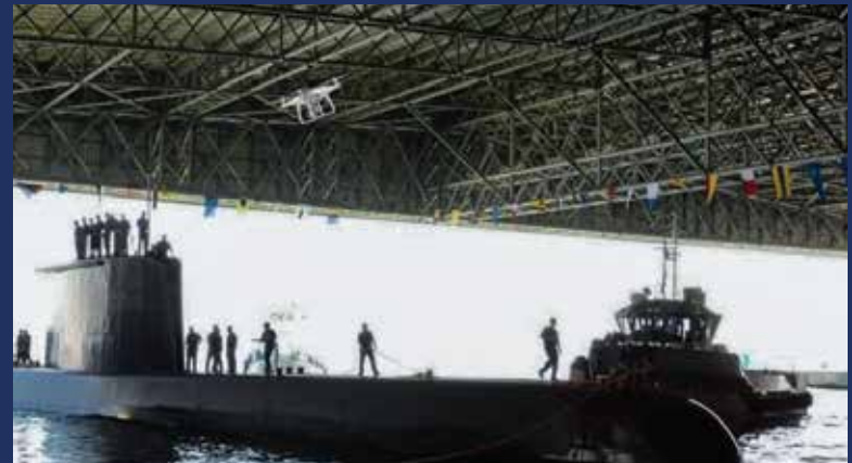
Submarines Hanger Project
