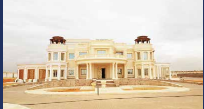
Fifth Settlement villas
